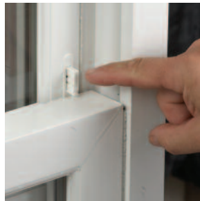
AAMA certified secondary vent locks securely limit how far the sash will open, allowing for worry-free ventilation.
