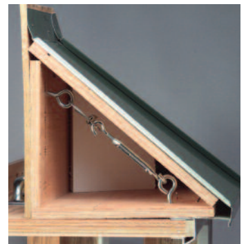
Concealed turn buckle cable support system ties back to the home for a secure, level window.
