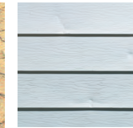
impact-damaged metal siding
