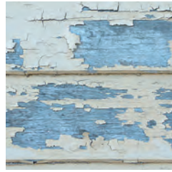
flaking painted wood siding
