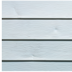
impact-damaged metal siding
