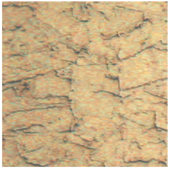
weather-damaged stucco
