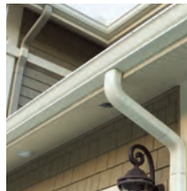
Elbows, Downspouts and Gutter
