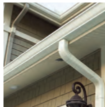
Elbows, Downspouts and Gutter
